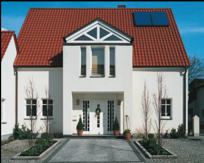
DHW system with flat-plate collectors
