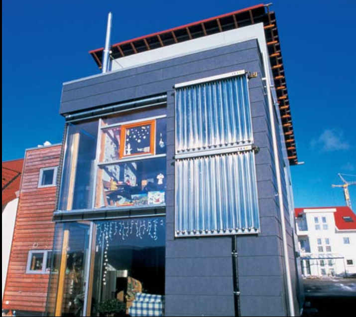
DHW system with vacuum tube collectors
