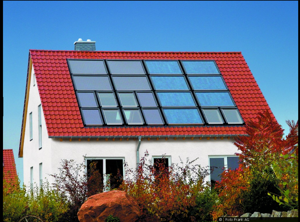
Left: combined solar thermal system for DHW and room heating support
